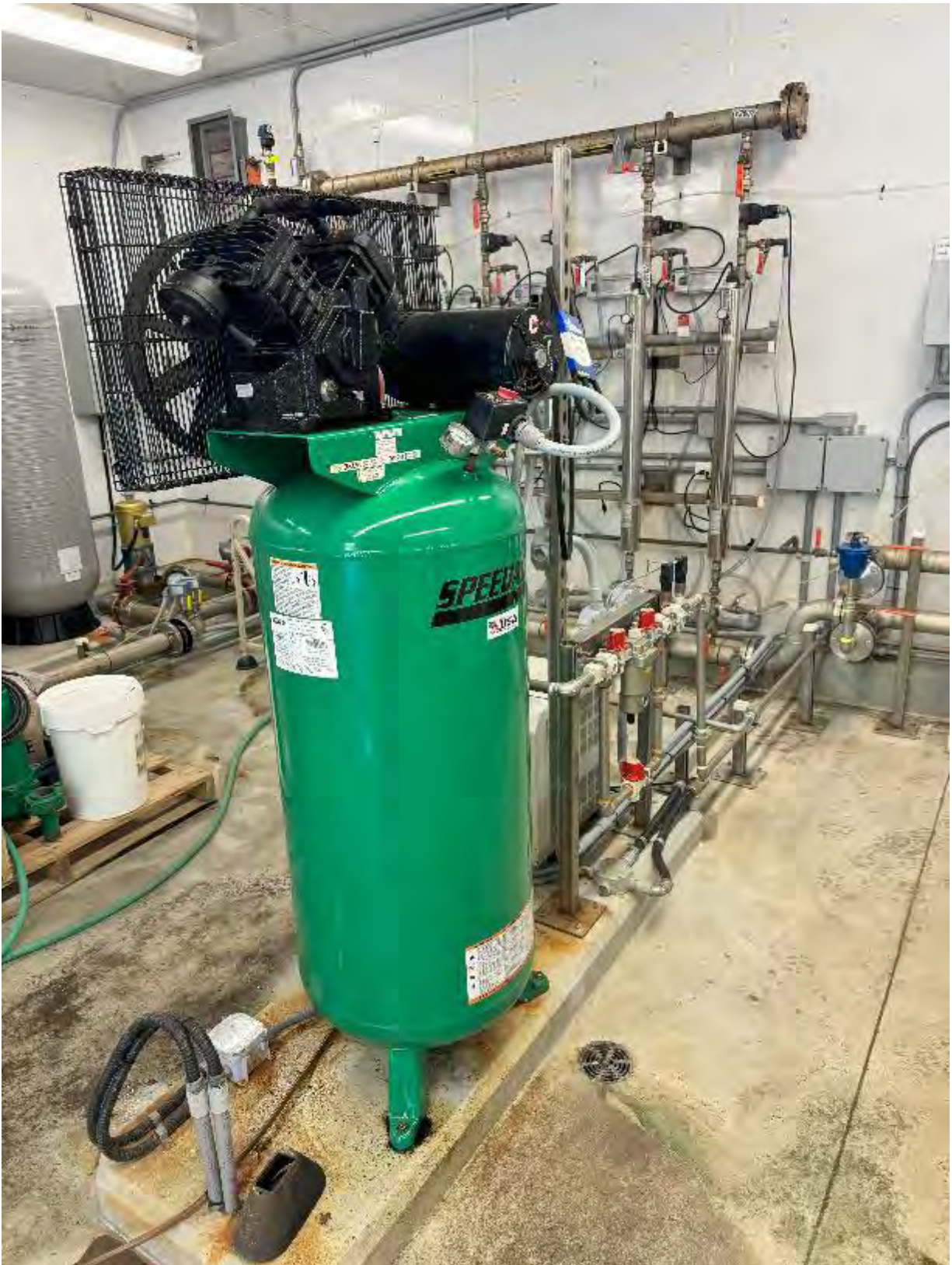
Photograph 6: Looking northeast towards compressor for membrane filters
